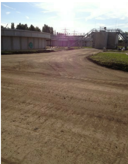
Un-surfaced simple RoadCem soil stabilisation, after two years use.
