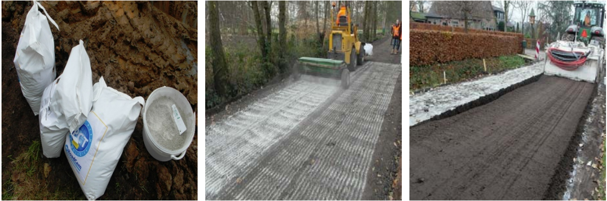
(a) Rc additive (b) Distribute by a spreader (c) Mixing Rc and in-situ sand
