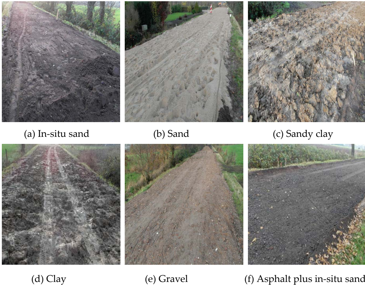
Figure 7.9 Preparation of the layers of soil materials
