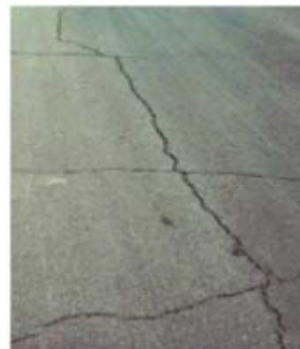
(b) Wide reflection crack
