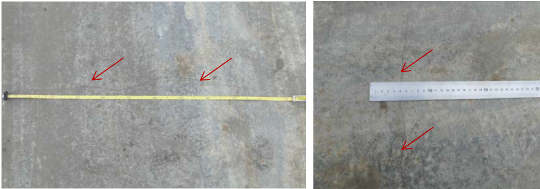
Figure 7.15 Observed cracks in stabilized sand section S-1
