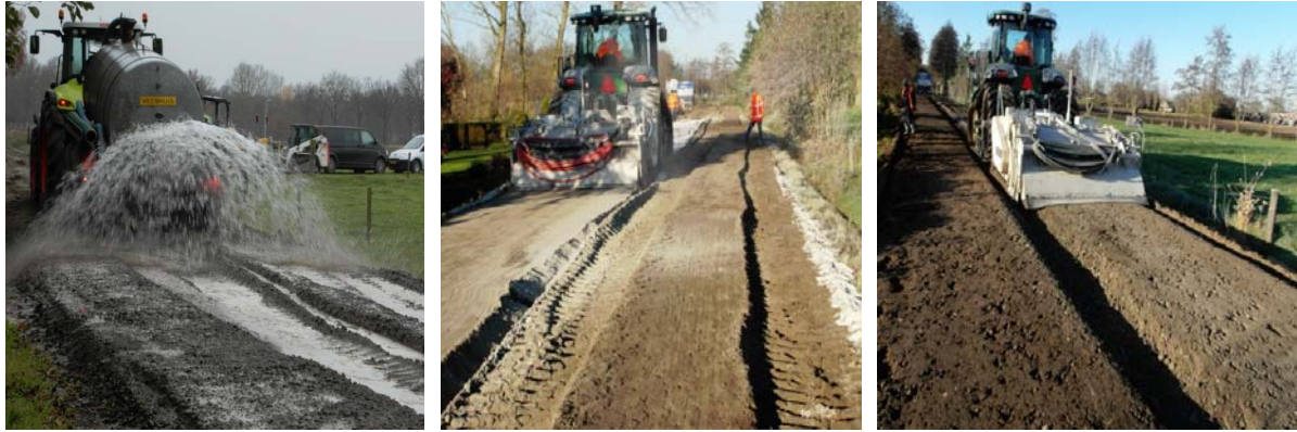
Figure 7.12 Adding water and wet mixing
