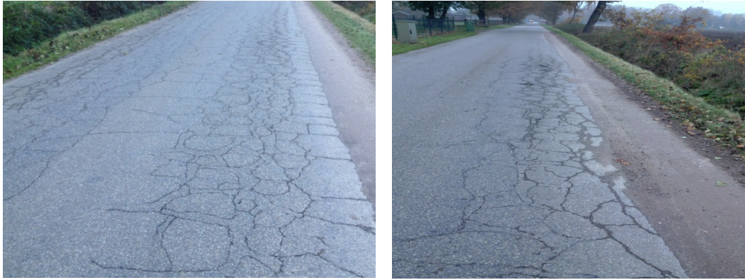
Figure 7.5 Observed distress in the existing asphalt pavement
