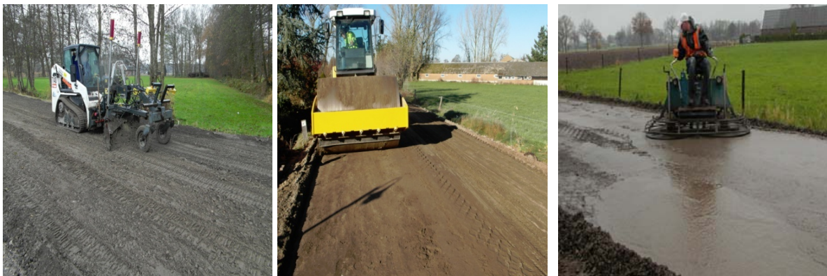
Figure 7.13 Levelling, compaction and polishing surface
