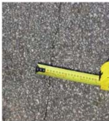
(a) Narrow reflection crack
