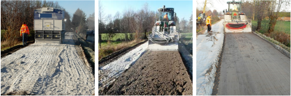
Figure 7.11 Applying cement and dry mixing
