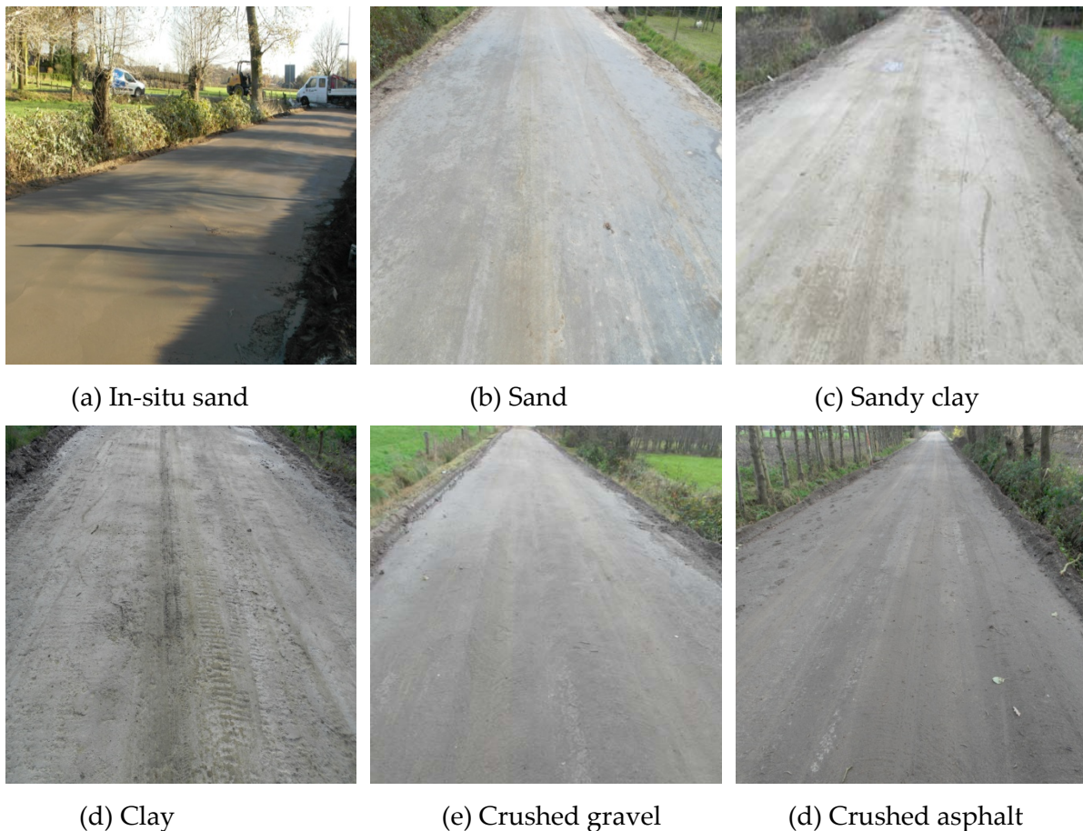
Figure 7.14 Cement stabilized base surfaces at 5 days after construction
