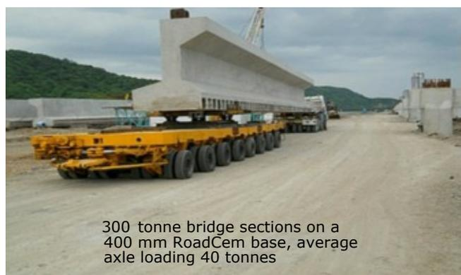
300 tonne bridge sections on a 400 mm RoadCem base, average axle loading 40 tonnes
