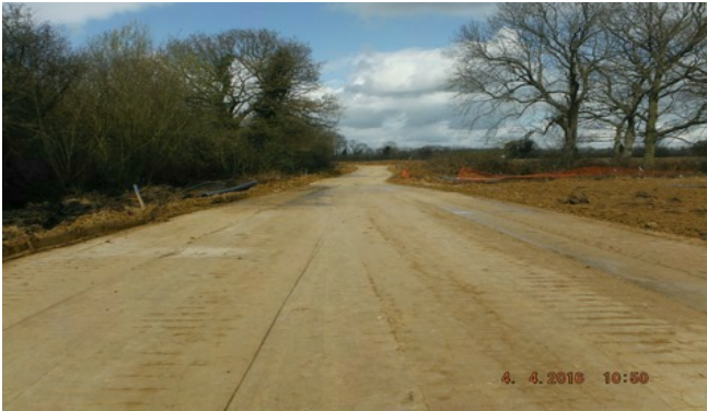
Temporary Haul Roads
