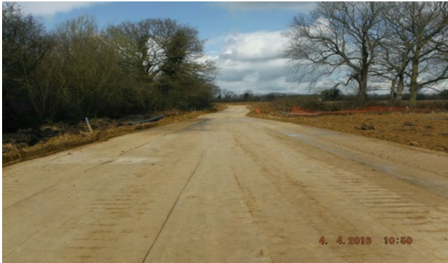
Temporary Haul Roads
