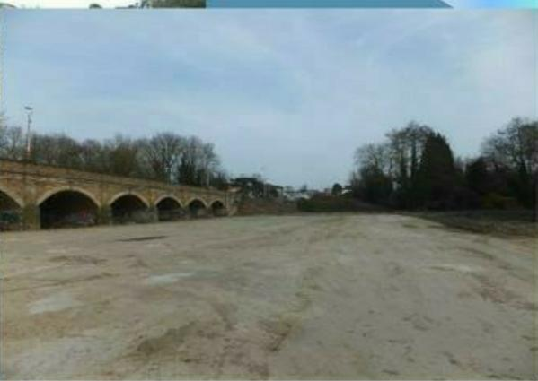
**10,000 m<sup>2</sup> RoadCem construction Platform to take heavy crane loadings of up to 80 tonnes /m<sup>2</sup>**
