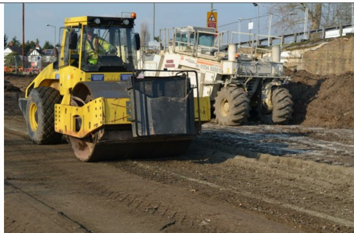
Pictures 2 & 3: Creation of piling platform at Walton on Thames Bridge over the river Thames (Costain & Atkins for Surrey CC).
