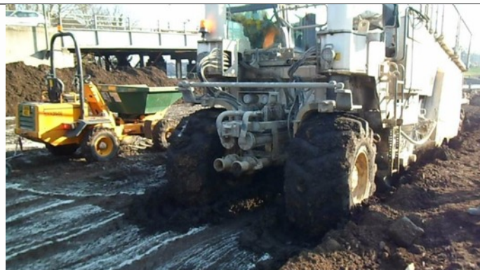
Pictures 2 & 3: Creation of piling platform at Walton on Thames Bridge over the river Thames (Costain & Atkins for Surrey CC).
