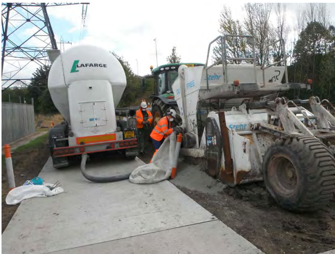
Plate 4 Incorporation of powercem and cement into topsoil
