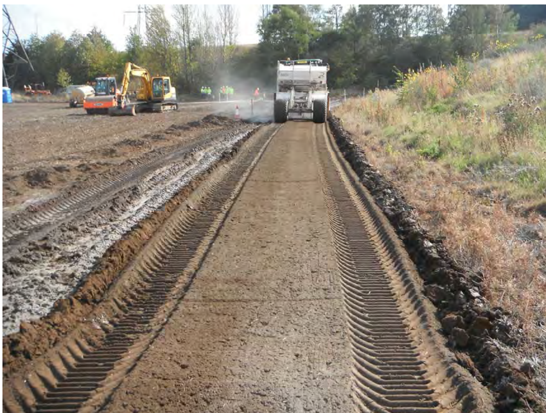
Plate 4 Incorporation of powercem and cement into topsoil
