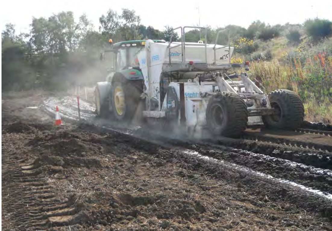
Plate 6 Incorporation of powercem and cement into topsoil
