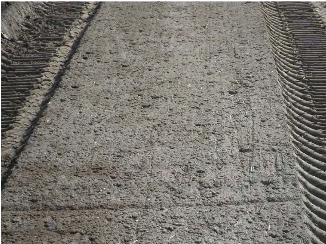
Plate 10 Prepared surface pre-compaction
