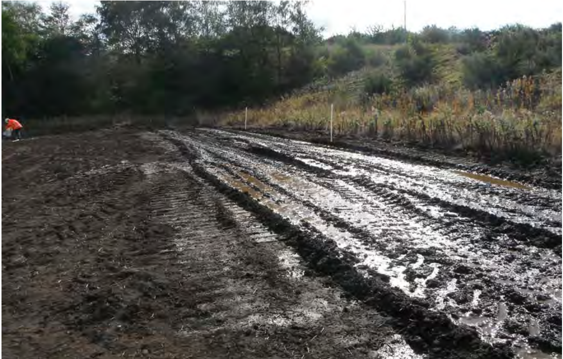
Plate 2 Application of powercem prior to incorporation
