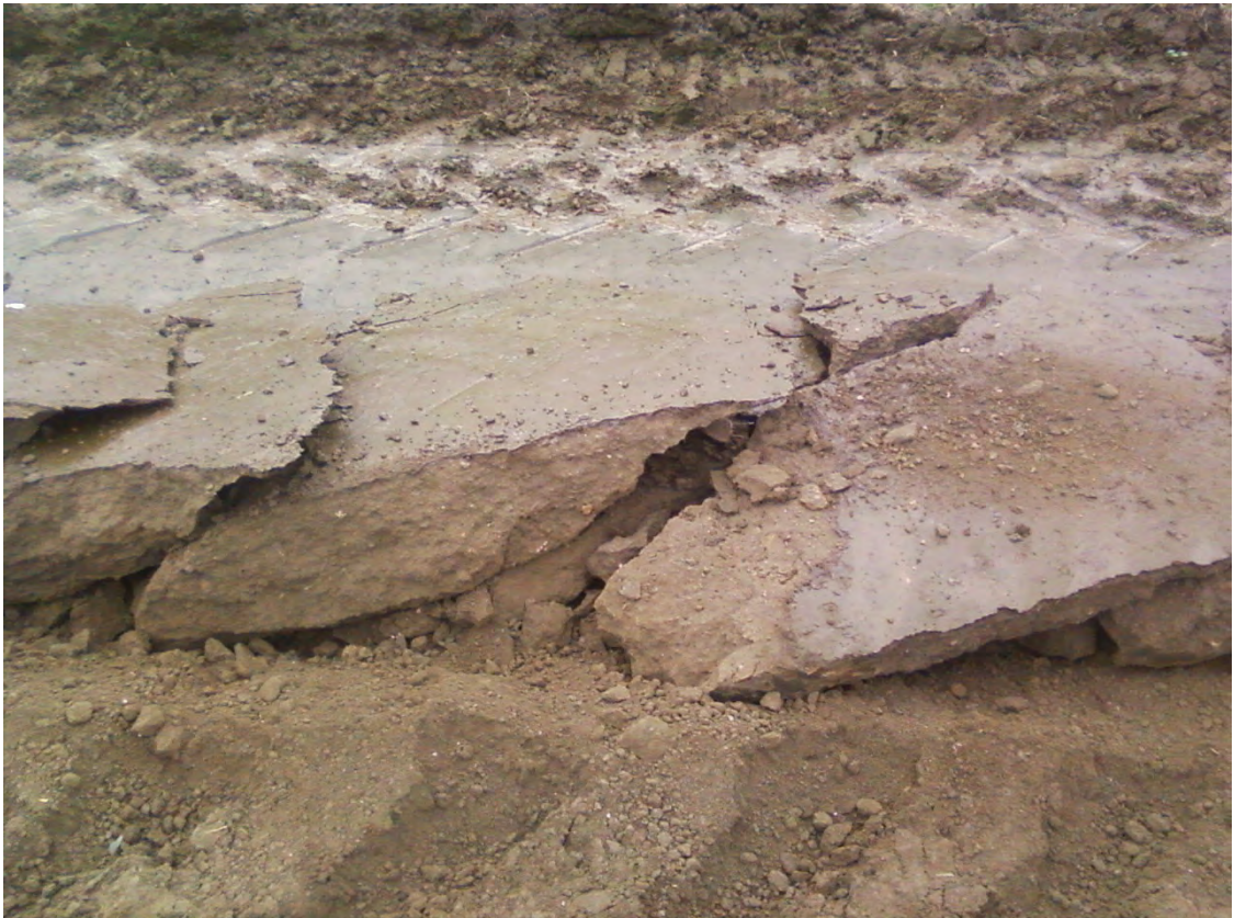
Plate 14 Track decompaction and cultivation
