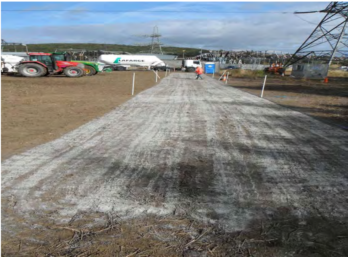
Plate 2 Application of powercem prior to incorporation
