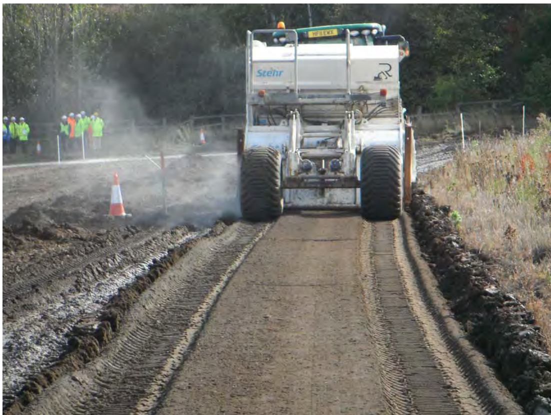
Plate 6 Incorporation of powercem and cement into topsoil
