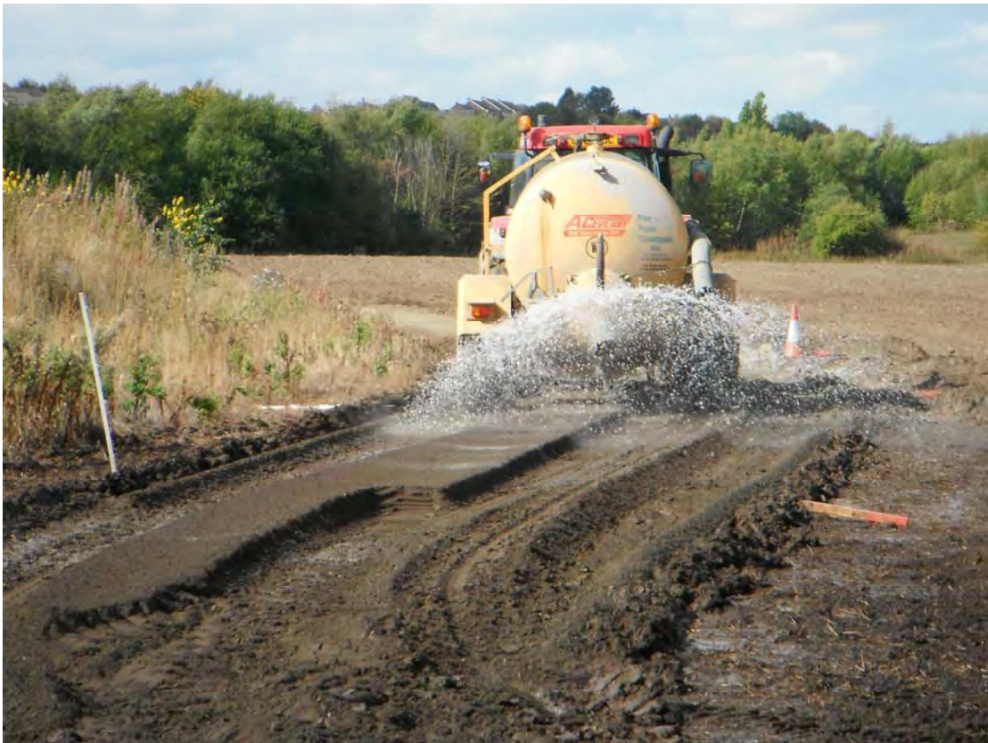
Plate 10 Prepared surface pre-compaction
