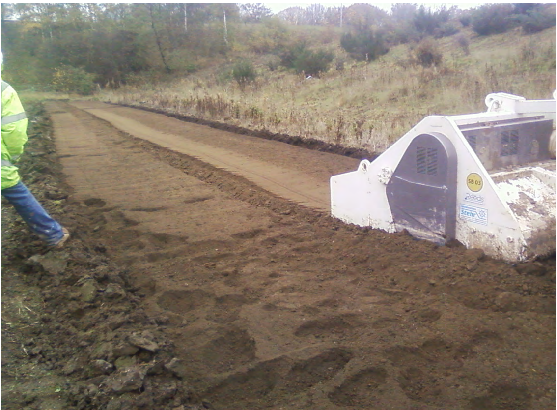
Plate 14 Track decompaction and cultivation
