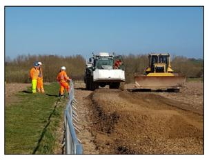
3.1 The removal process had created finely-tilthed topsoil where rotovation had been set to 300 mm depth. However, a mixed layer of topsoil and subsoil had been created along the upper part of the trial strip where rotovation had been to 500 mm. The eastern edge of the trial roadway had not been completely removed due to equipment breakdown<sup>1</sup>.
